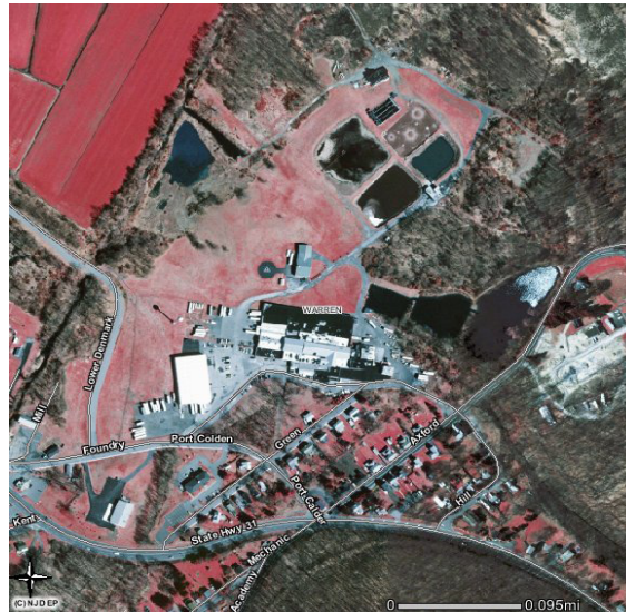
An aerial view of the Oxford Textiles site in Warren County, NJ (courtesy of NJDEP's iMap program).
