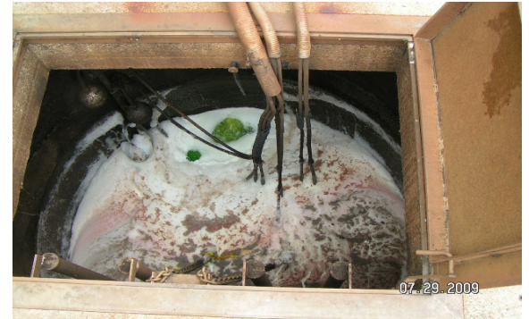
Leachate from the Kingsland Landfill.
