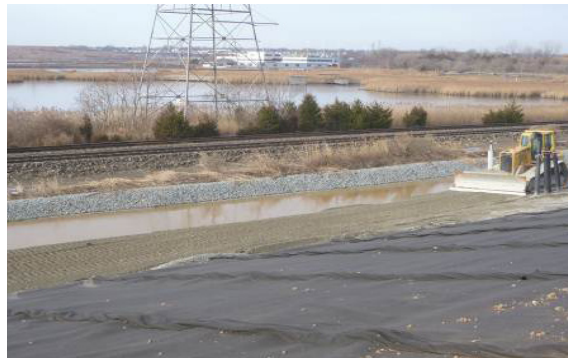
A view of the railroad tracks adjacent to the Avon Landfill.
