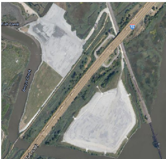
An image from Google Earth showing the landfills for Rutherford East and West.
