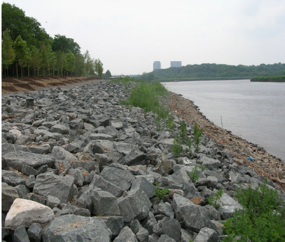
Summer 2008, at the newly restored and landscaped site.
